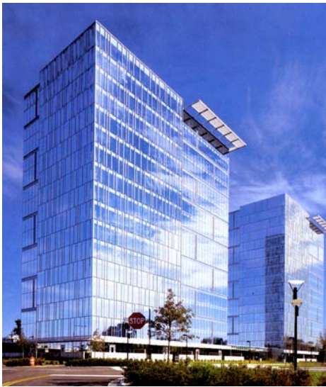
The LEED certified Reflections condominiums at the Bloomington Central Station near the Twin Cities International Airport is a good example of high density “green” building and site.
