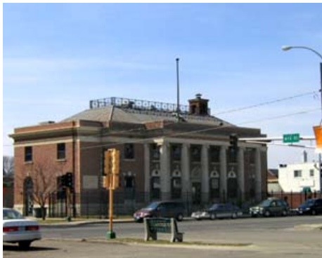
As one of the few landmark buildings in downtown Moorhead, the Rourke Art Museum in the historic Carnegie Library could serve as an anchor for a new Civic Campus.
