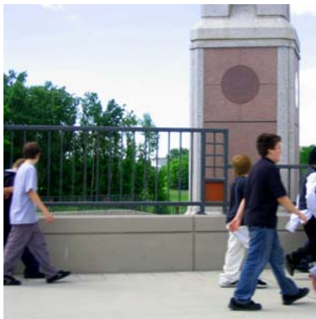
New Main Avenue Bridge over the Red River provides convenient pedestrian access between downtown Fargo and Moorhead.
