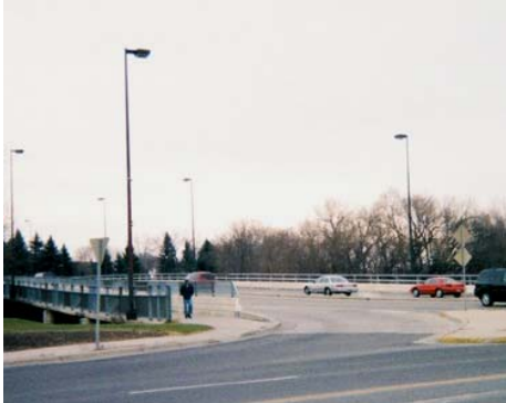
View of 1st Avenue Bridge looking towards Moorhead.
