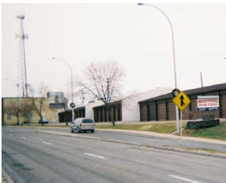
View of existing storage facility on Main Avenue in Fargo.
